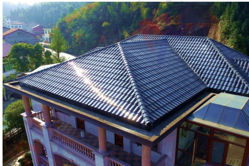
BIPV Roof: Solar roof tiles
